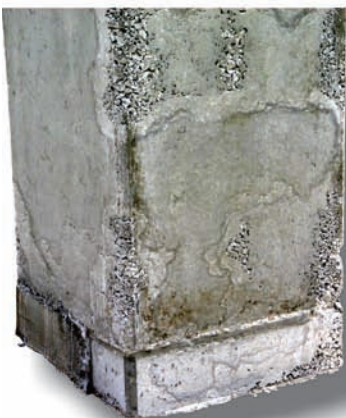
With high-cycle vibration in congested rebar
